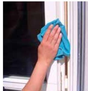
Every time you clean the surface, it is important to look for cracks of the paint films caused by hail or possible mechanical shocks that may allow water to penetrate in the wood underneath. Any time you notice such situations, you must intervene immediately with retouching.
