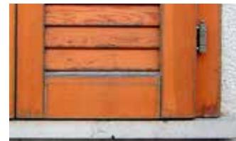
Check carefully the heads of the shutters and the horizontal surfaces where the first cracks on the paint film may appear
