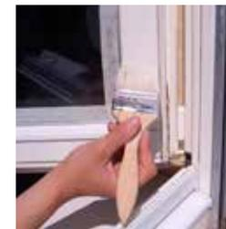
Clean the surface using water and dishwashing liquid.
